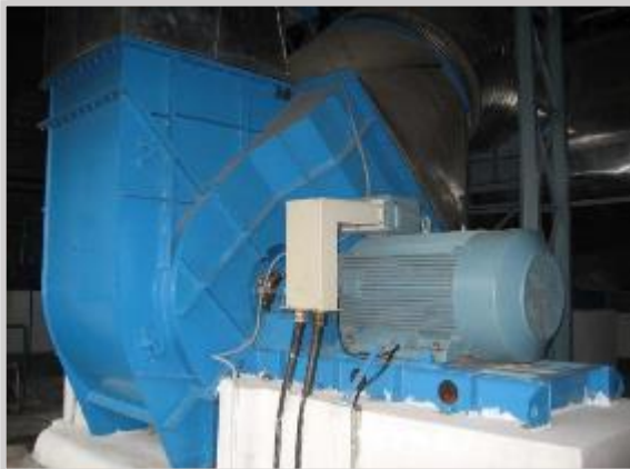
MVR Fan-Heart of the system
