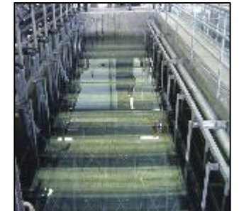
Membrane Bio reactor (MBR)
